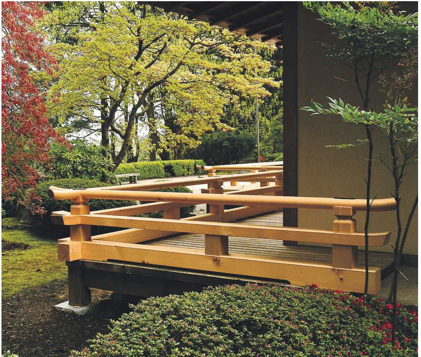
Photograph courtesy of Dale Brotherton – www.japanescarpentry.com; all other photographs by Michael Huntley
